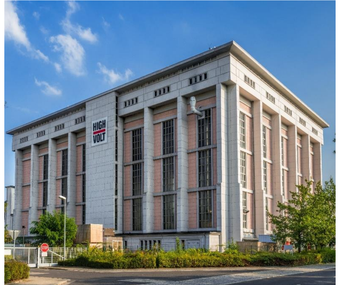
Large HV test hall (60 m x 47 m x 33 m)
